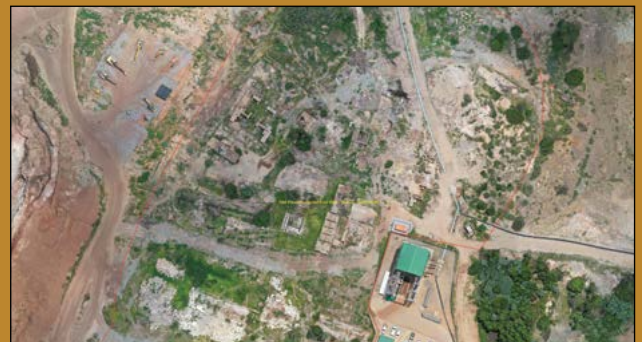
Old Plant Infrastructure remnants - Before rehab
